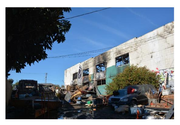
A single door-opening (created by removing concrete blocks from the wall) was present along the ground floor, at approximately the midway point (see below-circled). Fire and smoke damage was heaviest above the middle windows on the 1<sup>st</sup> and 2<sup>nd</sup> floors. (see photo below)
