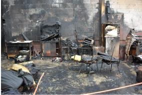
3. No floor level burn patterns were observed in the northeast section. Fire patterns indicate flames burned above floor level.
