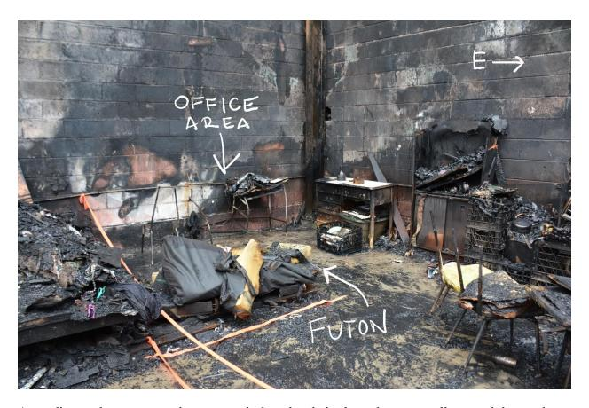
According to the occupant, there was a desk and a chair along the west wall, toward the south end of the office space. The metal frame of the chair was located. The backrest and seat were consumed. The only remains of the desk were heavily charred pieces of wood.
