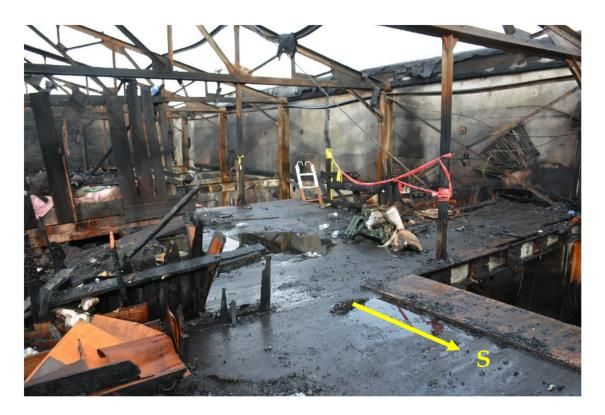
Overall, less damage was observed within the front (south) half of the warehouse, on both levels. Despite the collapse of the rear half of the second floor, investigators were able to observe burn patterns to be more severe on the undersides of the collapsed floor of the second floor, indicating more flame impingement from below.
