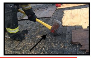
Use the back side of the axe for cutting, it seems counterintuitive but the flat side of the axe provides better "chopping" of roof materials and is less likely to bind into the roof.
