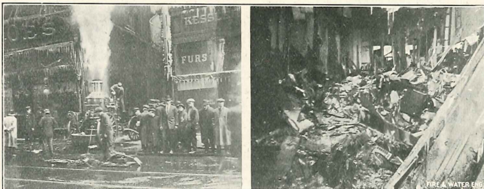
VIEWS OF ALOE OPTICAL CO. BUILDING, ST. LOUIS, AFTER FIRE.
