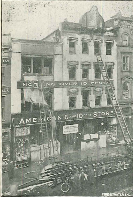
AMERICAN CO. BUILDING, WASHINGTON, D. C., AFTER FIRE.
