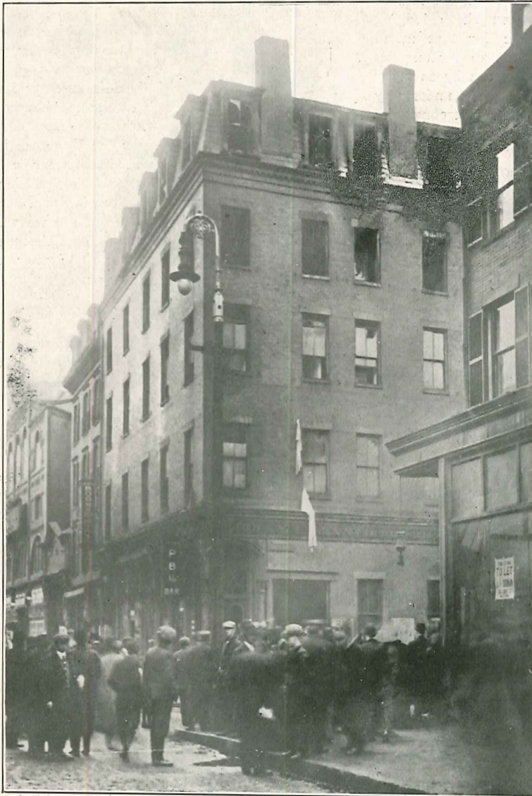
ARCADIA LODGING HOUSE, BOSTON, AS IT LOOKED AFTER THE FIRE. NOTE THE ABSENCE OF FIRE ESCAPES.
