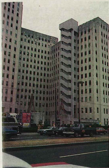
This outside fire escape was added to a New Orleans hospital when interior exits were found to be inadequate.
