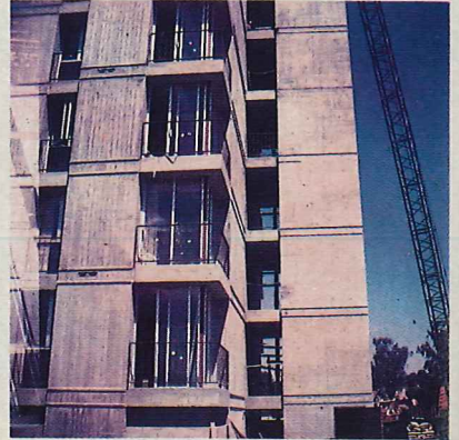
A California university installed this excellent exterior fire tower on dormitories.
