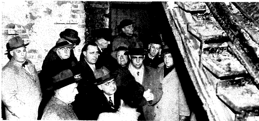
Members of Coroner's jury inspect stairwell where fire is said to have started
