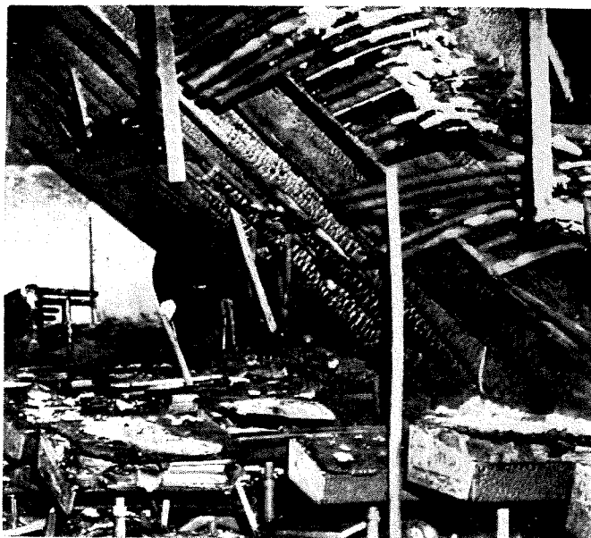
Roof collapse into classroom. Depth of char in portion of rafters indicates fire may have been burning for some time
