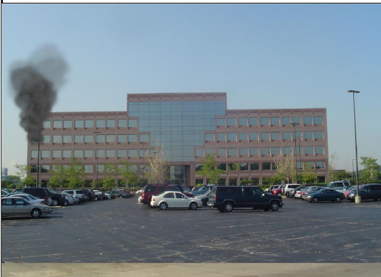
What is unusual about this smoke/fire condition from this construction type?
