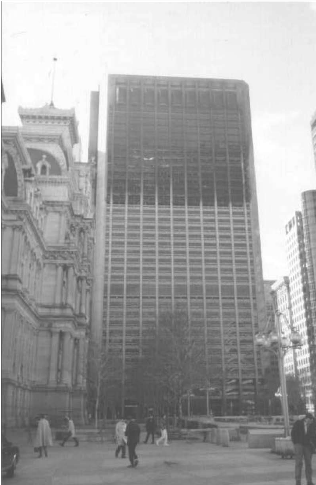
Exterior view of building looking south from City Hall Plaza.
