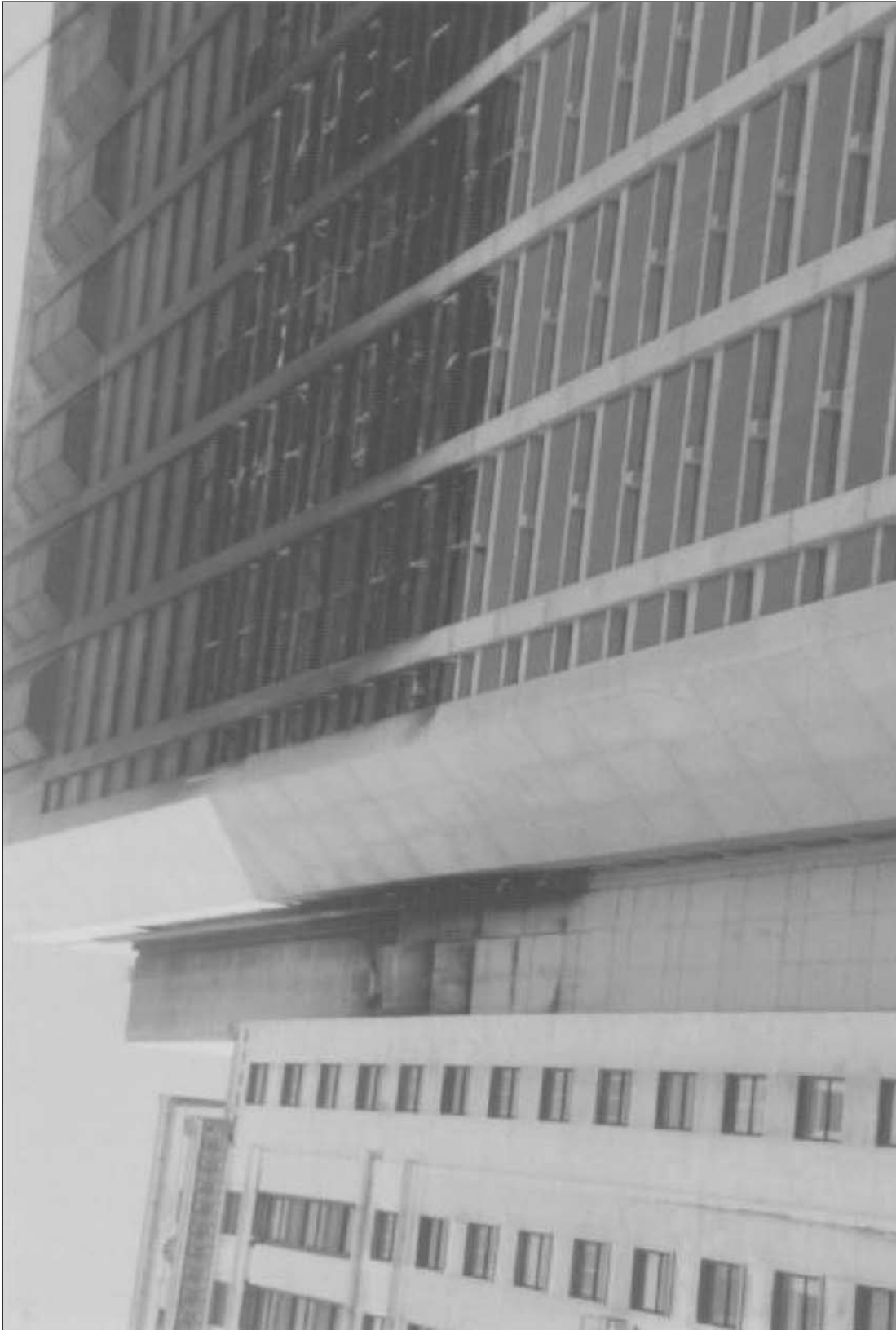
This stairway connected the One Meridian Plaza Building with the adjacent office building.
