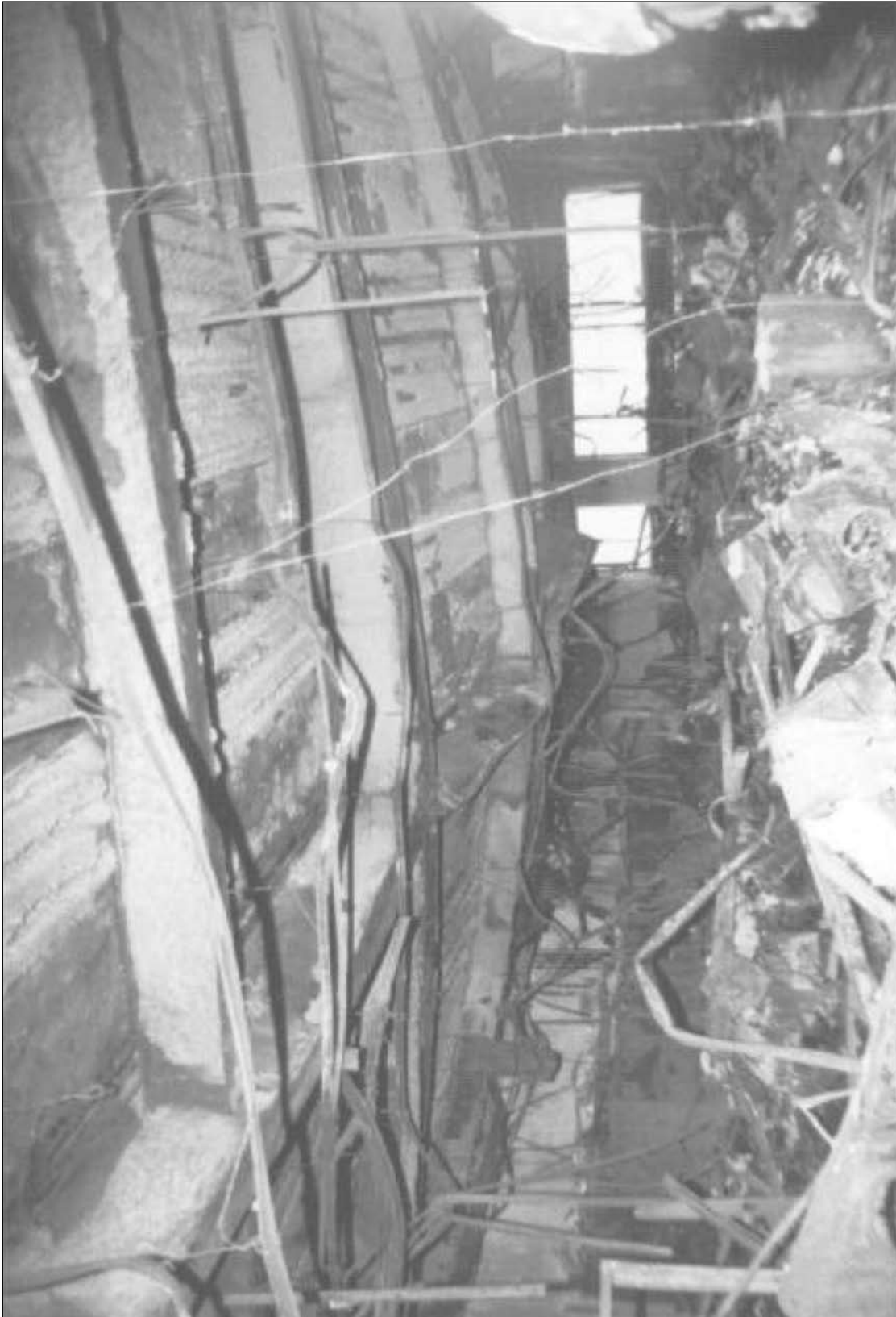
Here and in the next three photos are interior views of floor areas after the fire. Note the total consumption of the available fuel and sagging of the floor deck of up to three feet between columns.
