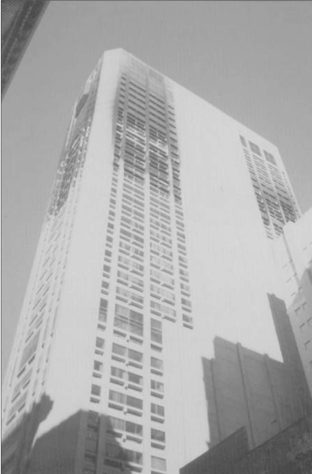
Exterior view of south side of building.
