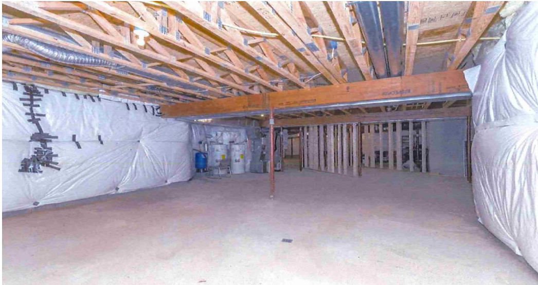
Figure 15: View of basement pre-fire from the Bravo/Charlie Corner.
