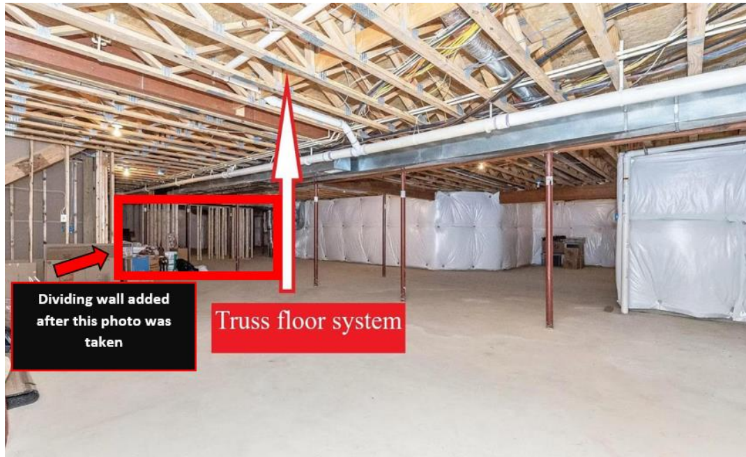
Figure 13: View of basement pre-fire from the Delta/Alpha Corner.
