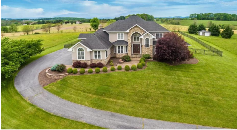
Figure 8: Aerial overview of structure.
