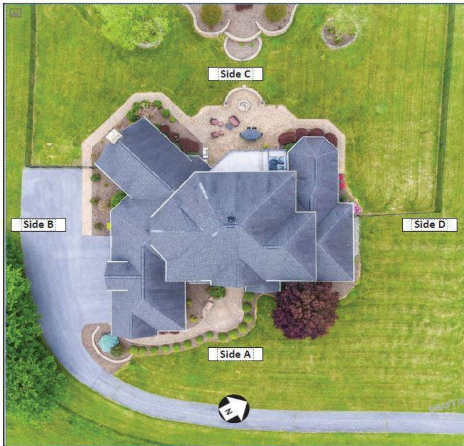
Figure 7: Aerial overview of structure.
