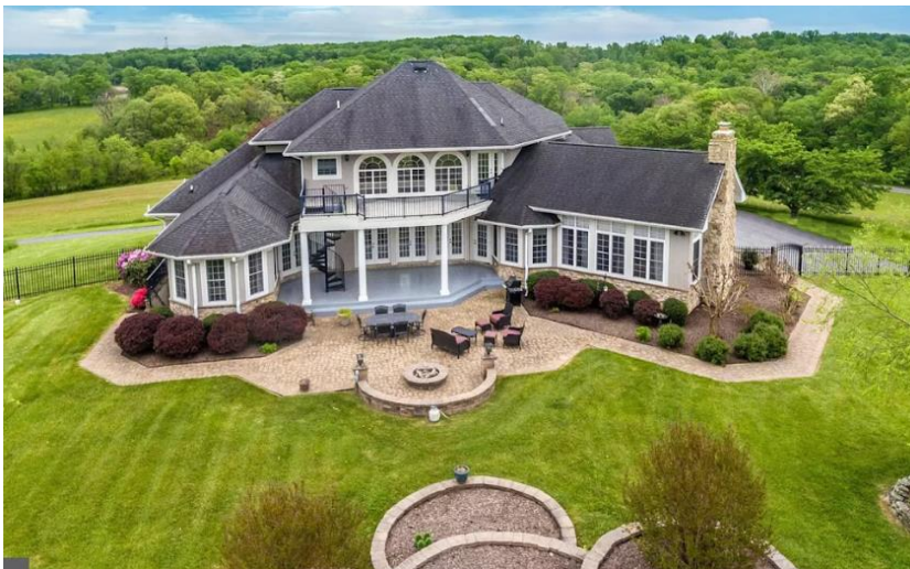
Figure 10: Side Charlie of the structure.
