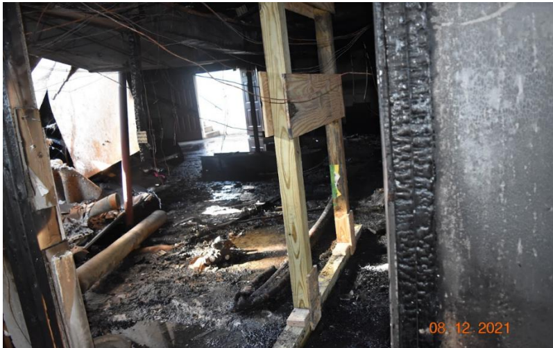
Figure 39: View of the distance and path from door in the interior basement wall separating the basement to the exterior basement entrance on Side Delta.
