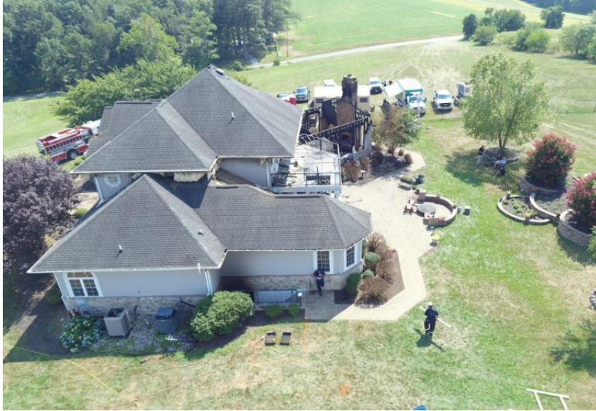
Figure 11: Side Delta with basement entrance.
