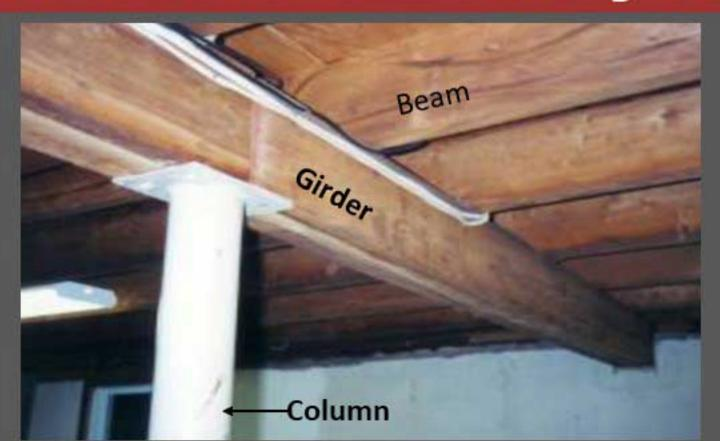
The term "hierarchy" as it relates to wood floor collapse indicates the seriousness of a collapse due to the failure of a bearing wall, column, girder, and beam.
