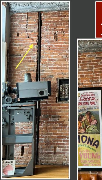
Both are important to watch, however a horizontal plane through the entire wall may be more likely to result in collapse with movement. Cracks occur in the weakest part of a wall, openings (typically windows and doors). Notice that these planes also may generate cracks.
