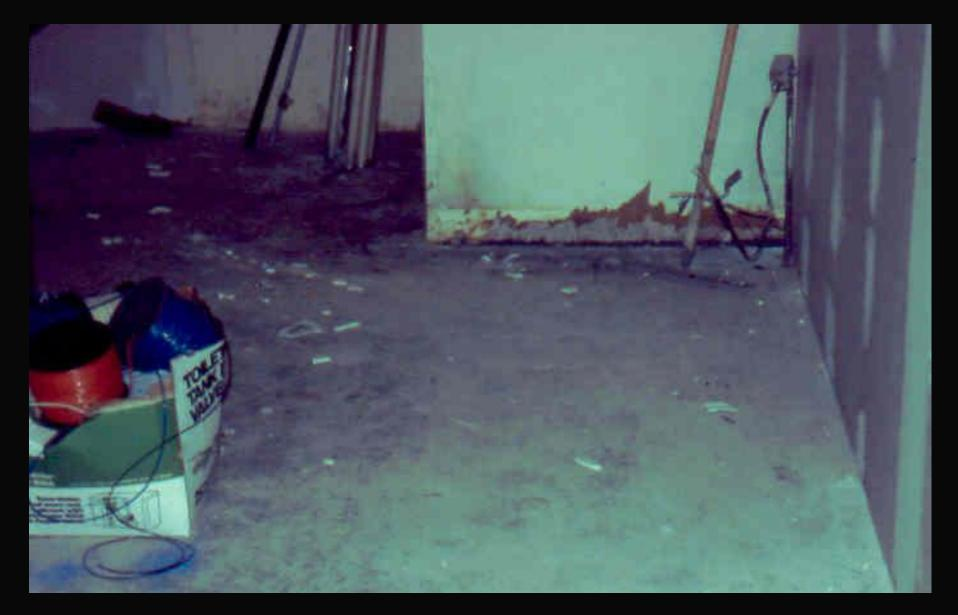
The alteration that added the concrete floor over the wood joists was accomplished by removing the finished and sub flooring from the area of the first floor. Wood furring strips were attached at or near the bottoms of each floor joist. The original subfloor was cut to fit between the floor joist bearing on the furring strips. The concrete was poured over the floor. This alteration added significant dead load to the structure.
