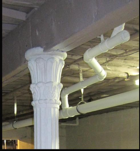
Additional photos of the wood beam crushing down over the tops of the cast iron columns. This condition existed at several column/beam connection through out the cellar.
