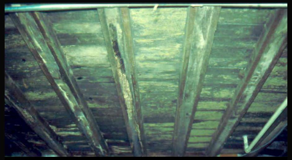
This photo depicts the condition of the first floor at the rear 1/2 to 1/3 of the floor area. Notice the floor joist are not visible to the full vertical dimension of the floor joists. There is also evidence of water damage to the floor joists and sub-flooring.
