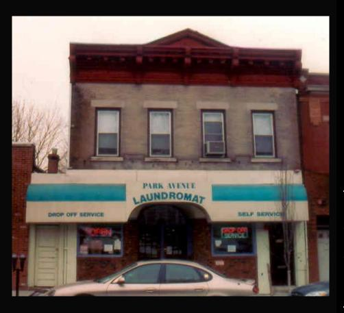
This building was constructed in 1911 of ordinary construction, has a full cellar. As with many buildings the structure was renovated over the life of the building. The following photos depict a renovation to part of the first floor that added significant dead load to the structure. The was building was occupied as a restaurant prior to being converted to a laundromat.
