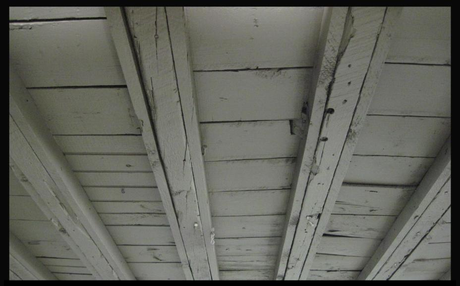
This is a later photo of the first floor at the rear 1/2 to 1/3 of the floor area. Notice furring strips nailed to the sides of each floor joist near the bottom of each joist.
