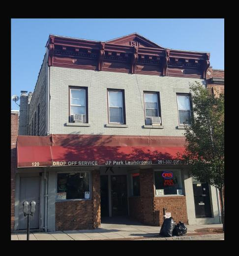
The building has a flat roof. The load bearing walls are the "B" and "D" walls. The floor joists and roof rafters span the "B" and "D" exterior bearing walls. There are column and beam assemblies that run from the "A" wall to the "C" wall, the column and beam assemblies support the floors. The photos will depict conditions that were photographed over the period of several years.
