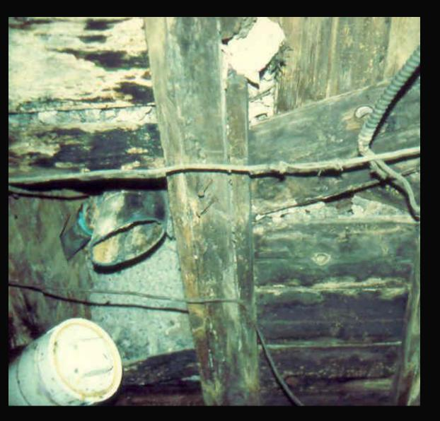
The concrete poured over the wood joist floor is obvious in this photo where the plumbing DWV pipe passed through the floor.
