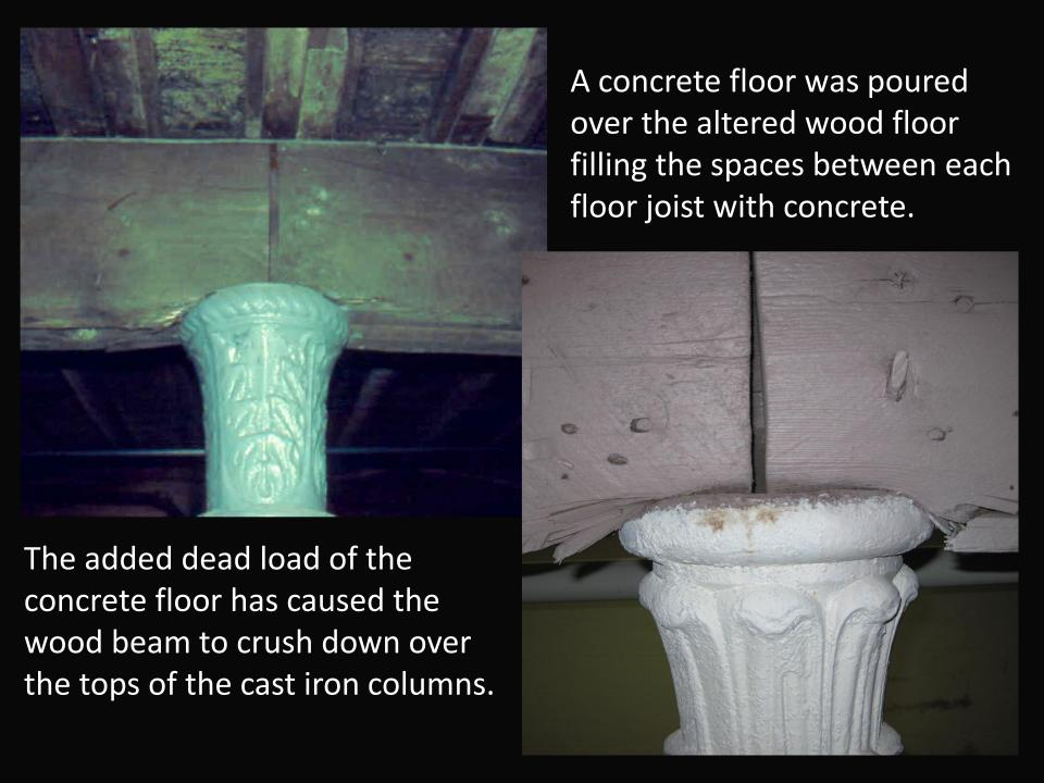
Another photo of the wood beam crushing down over the tops of one of the cast iron columns. Deterioration of the wood likely from water damage is also visible in this photograph.
