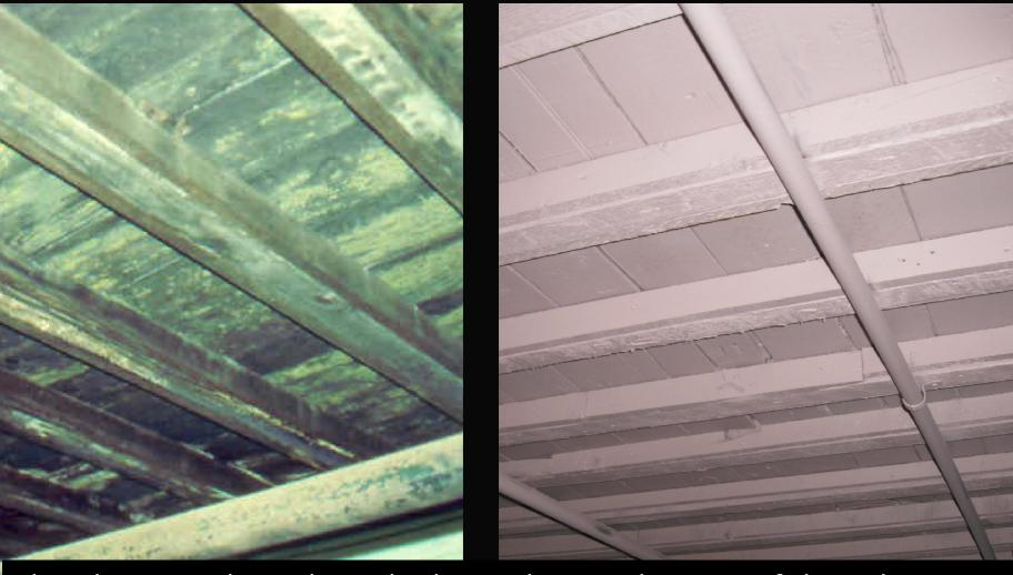
The photo on the right is the later photo, take note of the subflooring material, the subflooring material was removed from the original floor, cut into 14" to 14.5" lengths and placed on top of the furring strips between each floor joist.
